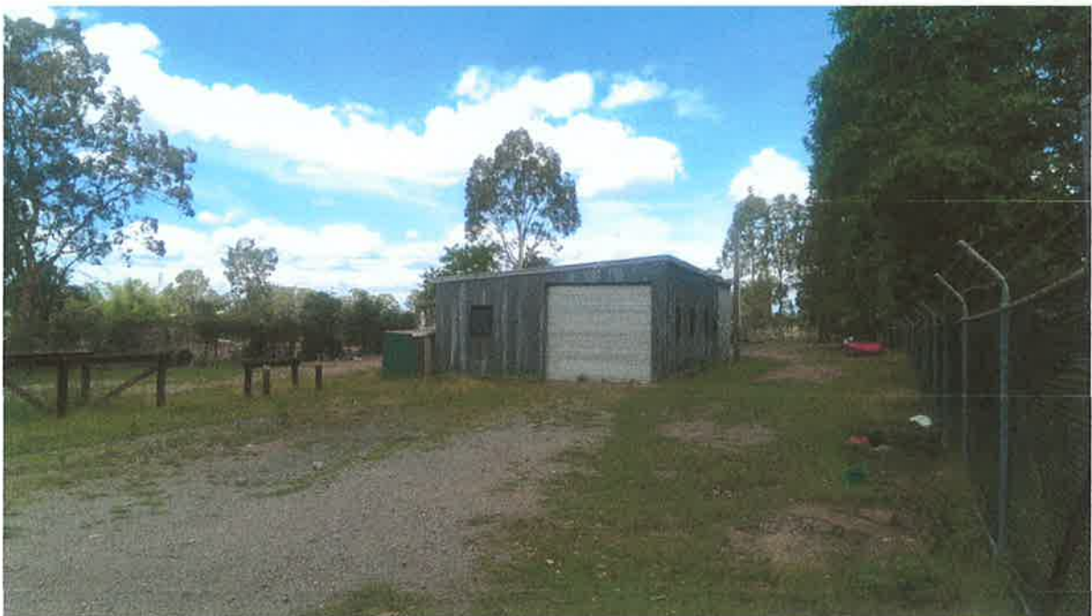
Corrugated steel shed on slab – the only remaining structure on site. Note - power pole adjacent to south west corner of shed.
