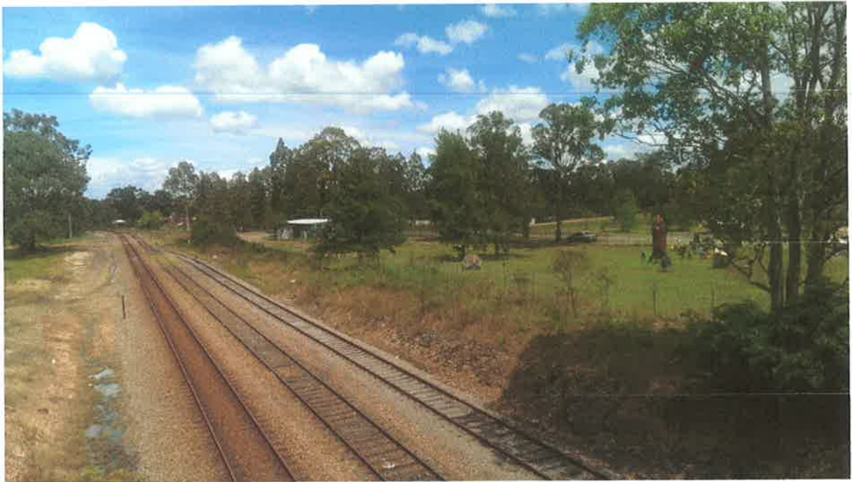
Site from Paterson overhead pedestrian foot-bridge (looking south)
